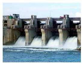
The amount of electricity generated from each power plant depends on the quantity of the flowing water and the height it falls from the reservoir to the turbines.
